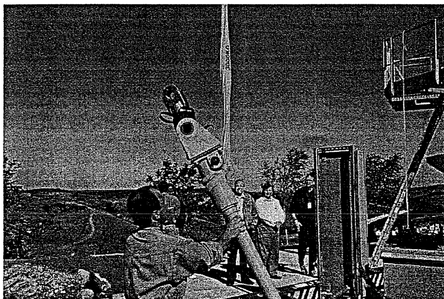
Figure 124 – Slings and positioning the elevation jack
