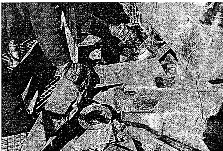
Figure 126 – Positioning the elevation jack
