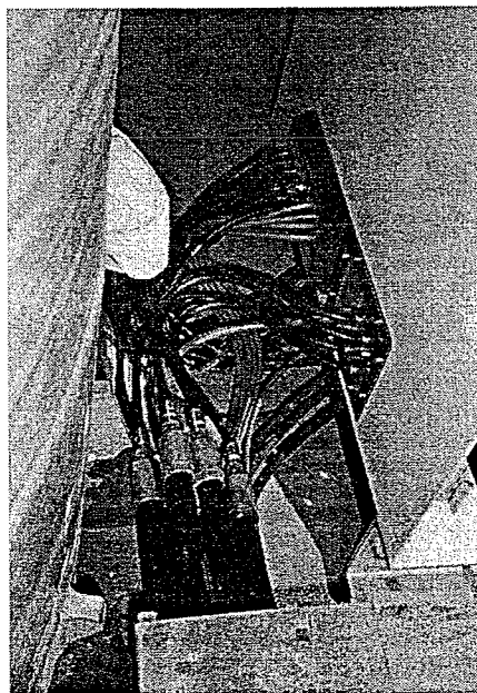
Figure 155 – Cable entry into the outdoor rack (optical fibre version)
