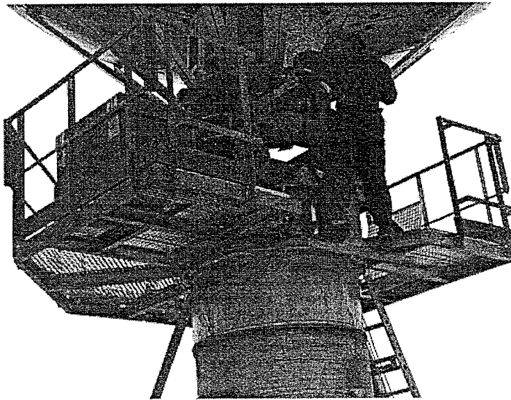
Figure 136 – Guiding the reflector and fitting the bottom trunnion
