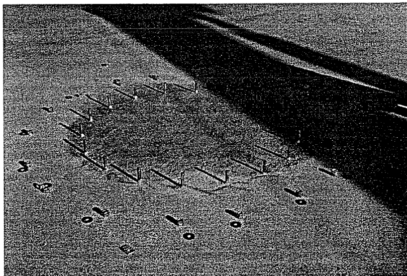
Figure 115 – Anchor studs, nuts and washers
