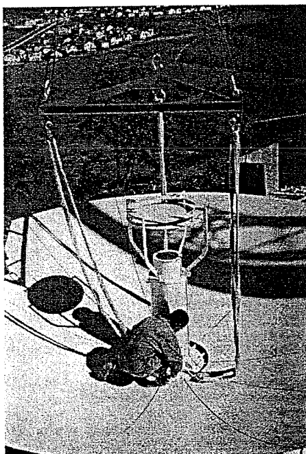
Figure 133 – Slings the hub/reflector assembly
