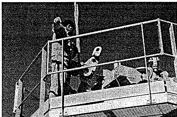
Figure 125 – Passing the jack through the platform
