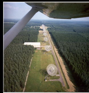
Westerbork synthesis radio telescope, single 25-m antenna is used for tracking experiments
